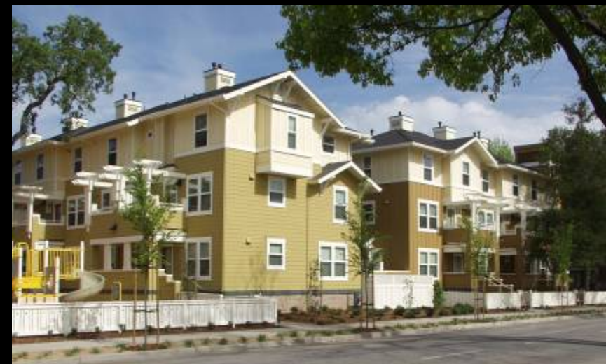
Courtyard above parking garage
