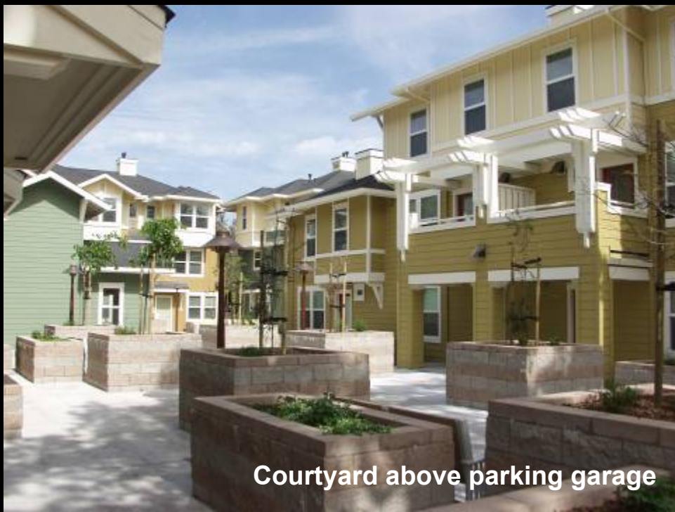
Porches with stoops rise to the lid above the parking garage.
