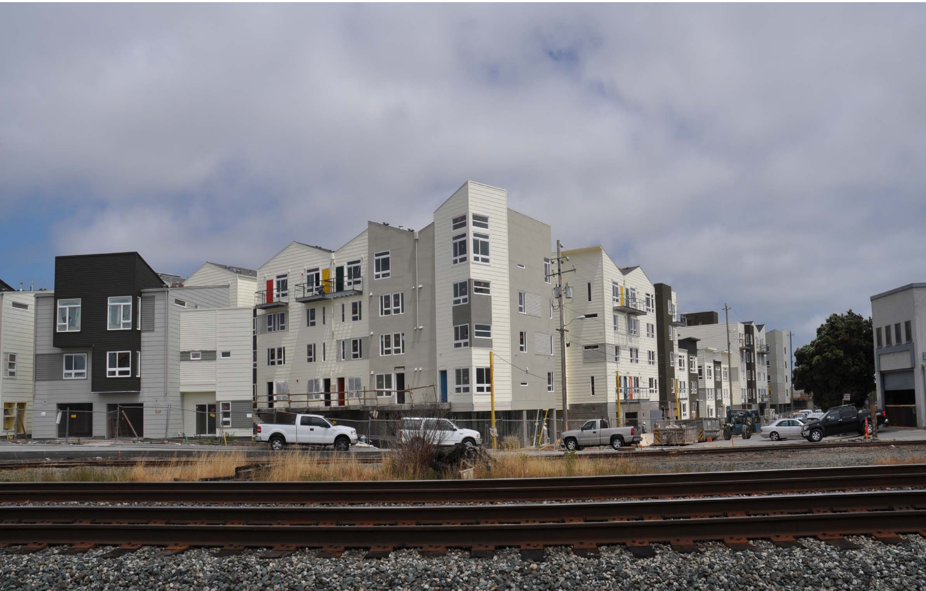
Project During Construction
