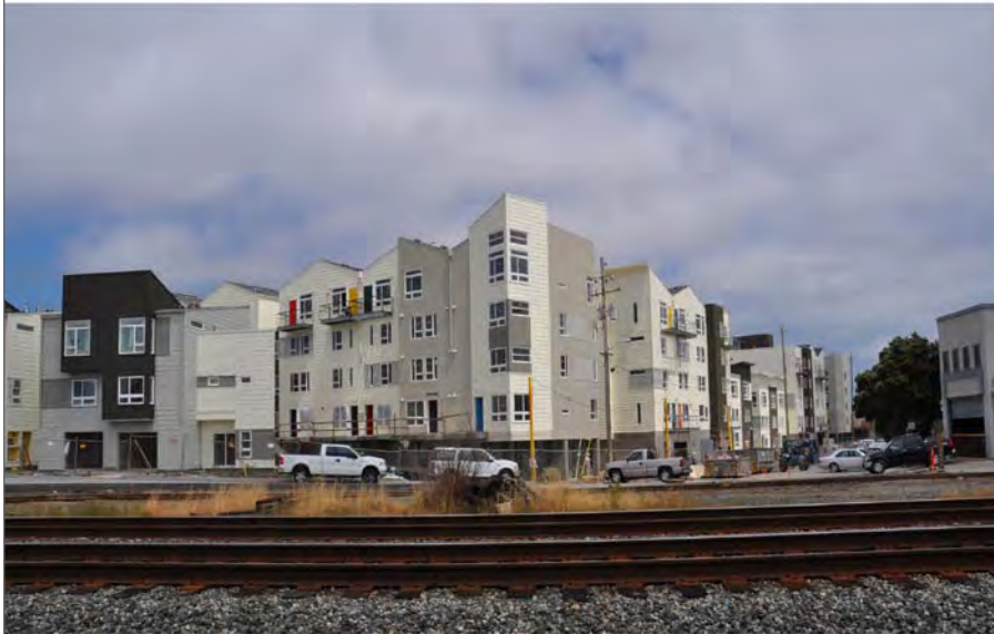
Project During Construction
