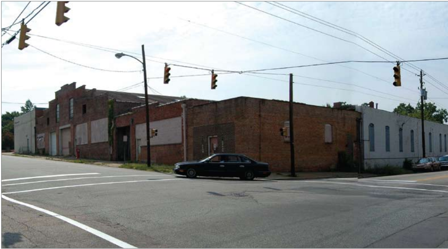
Stone's Warehouse: View from East and Davie streets.
