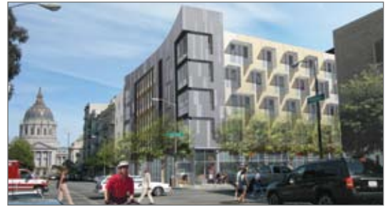
Parcel G, San Francisco: David Baker + Partners, Architects. Mixed used development including pedestrian-friendly ground floor commercial space.
